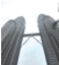
Fig. 13 A two-hinge arch supporting the Skybridge 6
